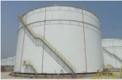
Storage tank annular plate and chime
