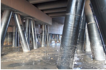
Pipe racks and structural steel
