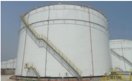
Storage tank base
