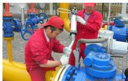
Field joints and fittings
