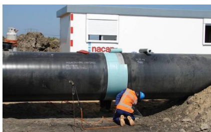
Buried pipeline field joint
