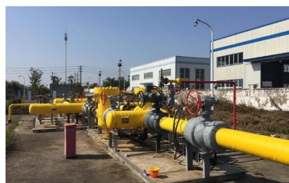
Coating repair on buried lines
