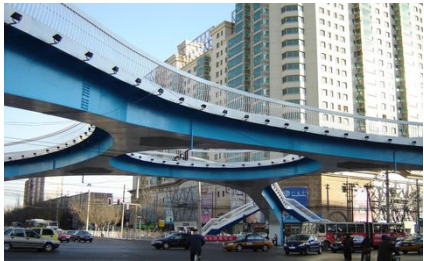
Bridges and exposed structures
