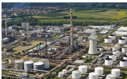
Process plant in direct sun
