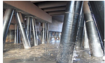
Pipe-rack utility lines
