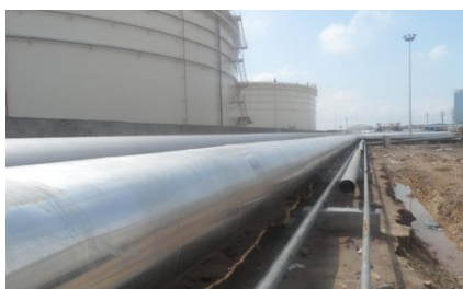
Buried pipeline construction
