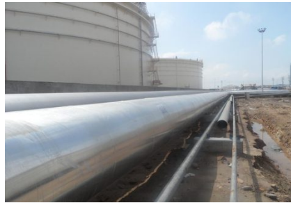
Buried pipeline construction
