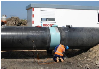
Field joint wrapping
