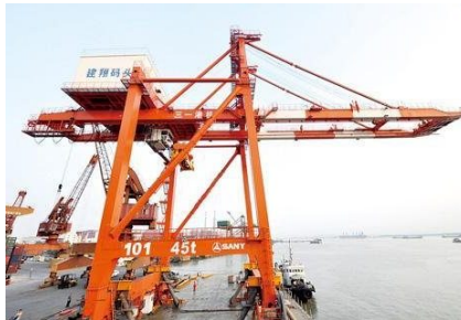
Port and terminal steelwork
