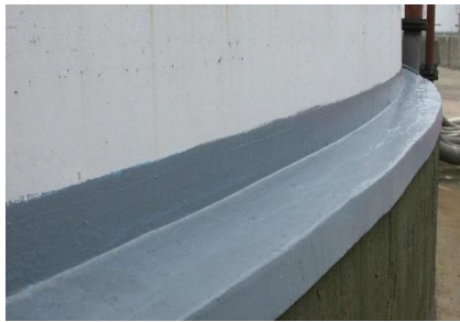
Completed tank edge system
