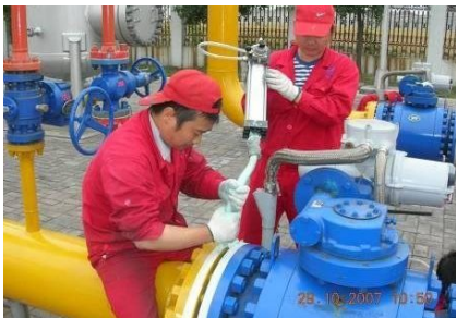
Valve chamber before wrapping
