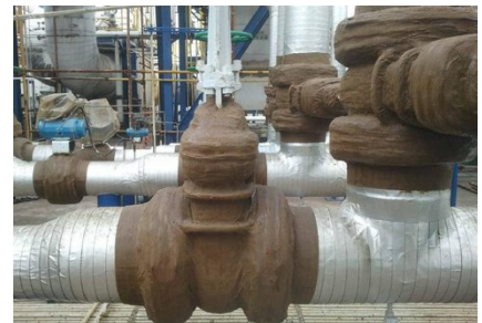
Completed valve and flange system
