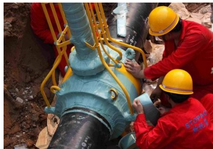
Wrapping in progress
