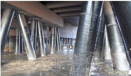
Exposed pipe rack
