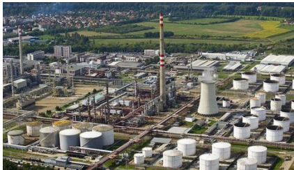
Process plant in direct sun
