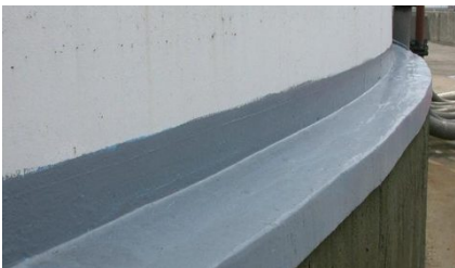
Tank base preparation
