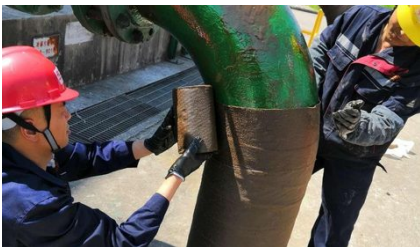
Chime detail build-up
