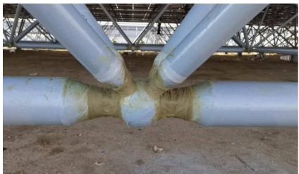
Overhead steel details
