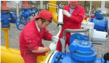
Profiling a valve body
