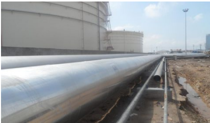
Buried pipeline construction
