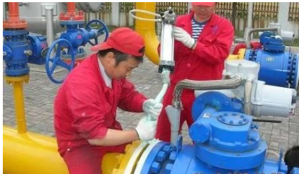
Field joints and fittings
