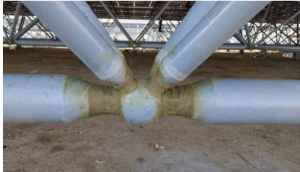
Structural steel connections
