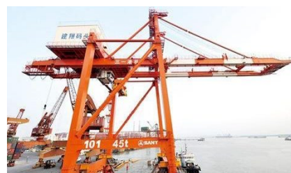
Port and terminal steelwork
