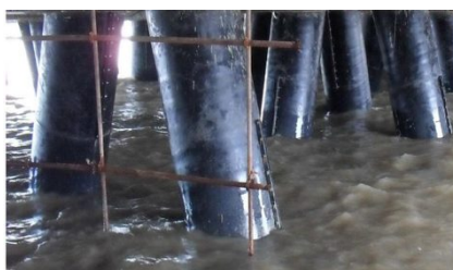
Steel pipe piles in water
