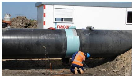
Field joint profiling
