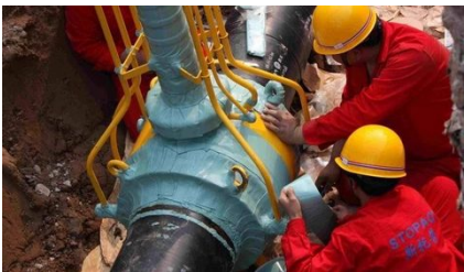
Valve and pump bodies
