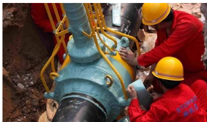
Valves, pumps and fittings
