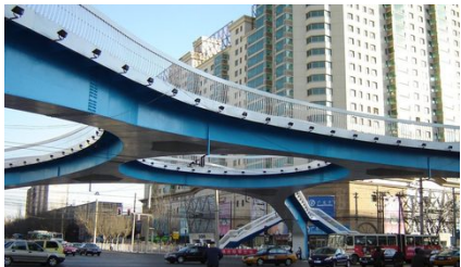
Exposed structural steel
